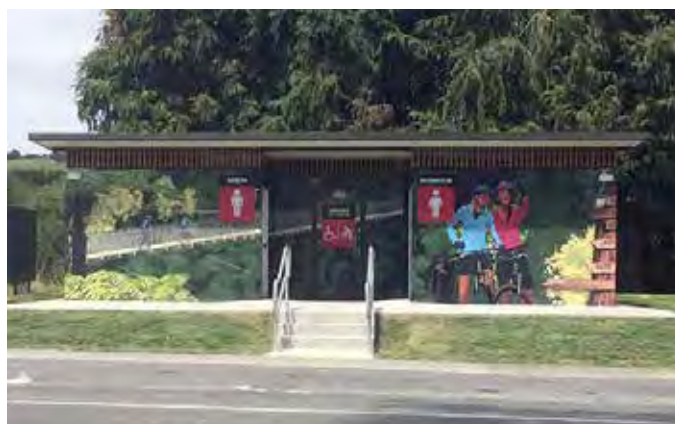
BENNEYDALE PUBLIC TOILETS
