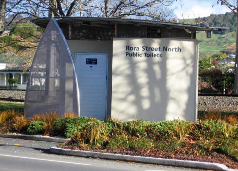
Rora Street North Public Toilets
