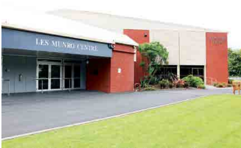
CHANGEOUT: Renaming the former Waitomo Cultural and Arts Centre to the Les Munro Centre is complete. Once renovations are finished, the centre will be officially reopened by Mr Munro's family in April.
