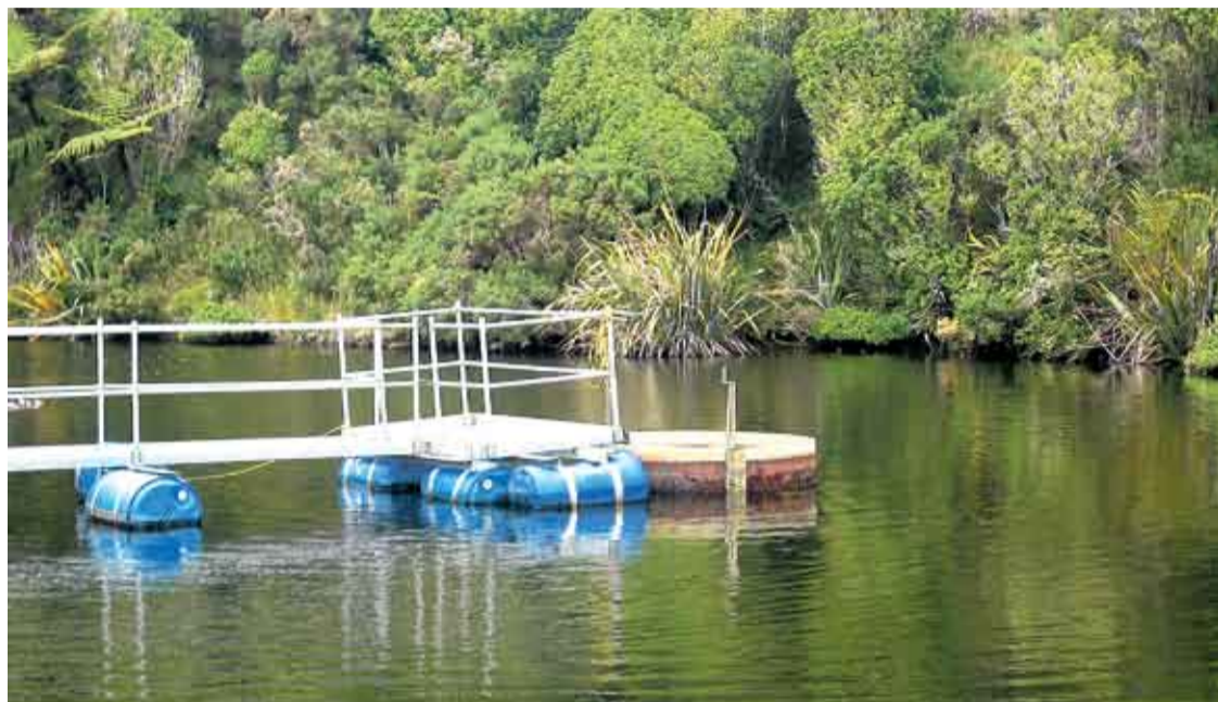
WATER SOLUTION: Waitomo District Council has approved the construction of a new dam in Mokau which will double the capacity of drinking water for residents. The existing dam (above) holds 10,000 cubic metres of water. PHOTO SUPPLIED
