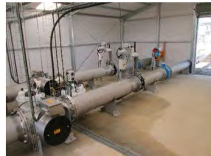
Wastewater Treatment Plant Bulk Lime Silo project has replaced the lime dosing hopper and dosing system, pipework is installed and SCADA integration complete. Dosing will minimise potential health and safety issues.
