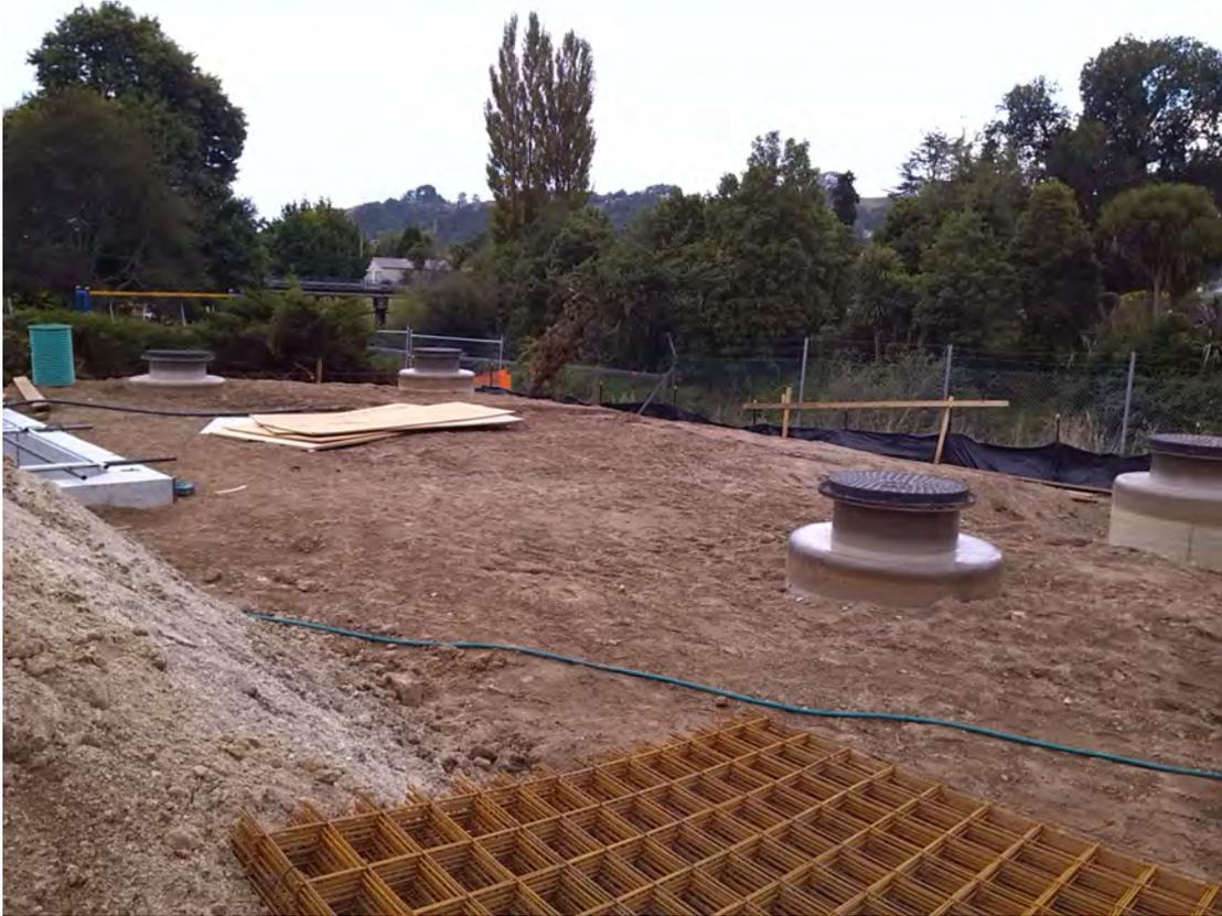
**Figure 2: Tanks after backfilling operations**
