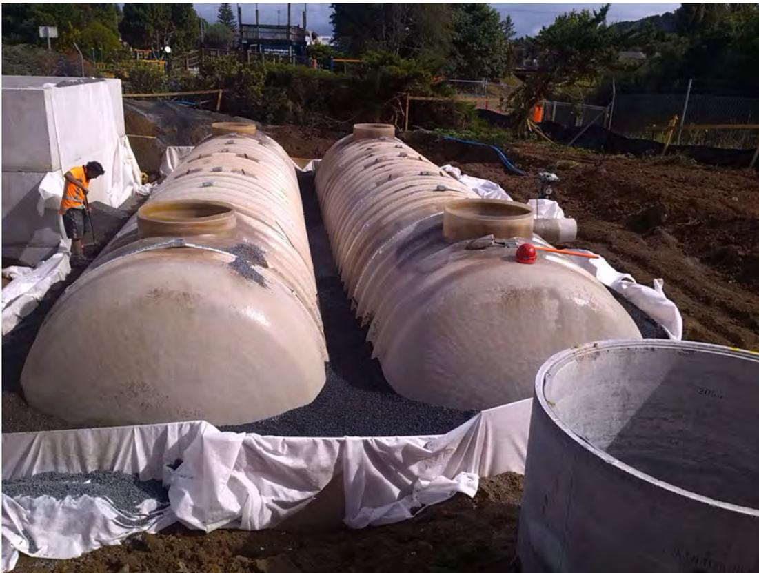
**Figure 1: Tank installations during backfilling operations**
