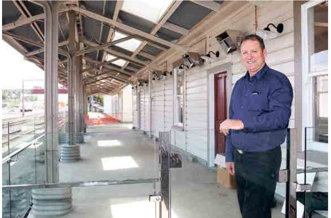
OPEN TO VIEW: Waitomo mayor Brian Hanna (outside the Te Kuiti railway buildings) and councillor Lorrene Te Kanawa (below, outside the relocated Te Kuiti Community House) are proud to finally welcome the community inside the recently renovated properties.
