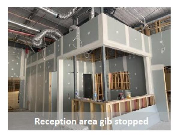
3.3 Internal framing for the amenities area has been completed and the interior wall separating the gymnasium area from the indoor playing courts (Gridline E wall) now lined.
