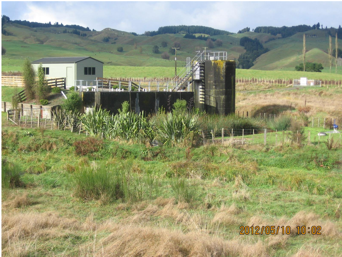
Benneydale Wastewater Treatment Plant
