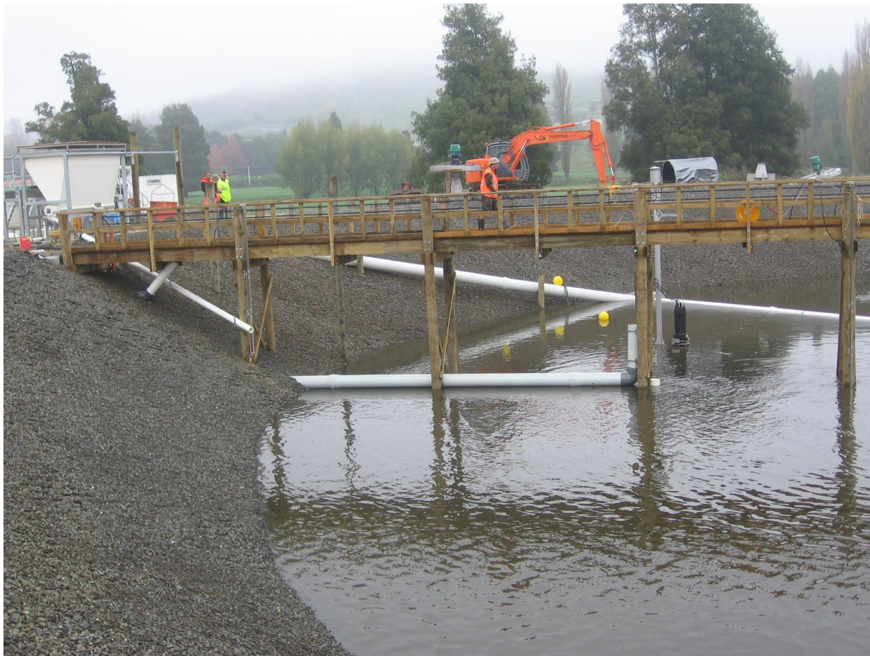
Fig 8.7 New Reactor April 2013
