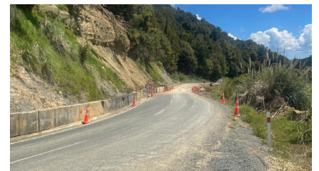
Pukerimu Road cleared
