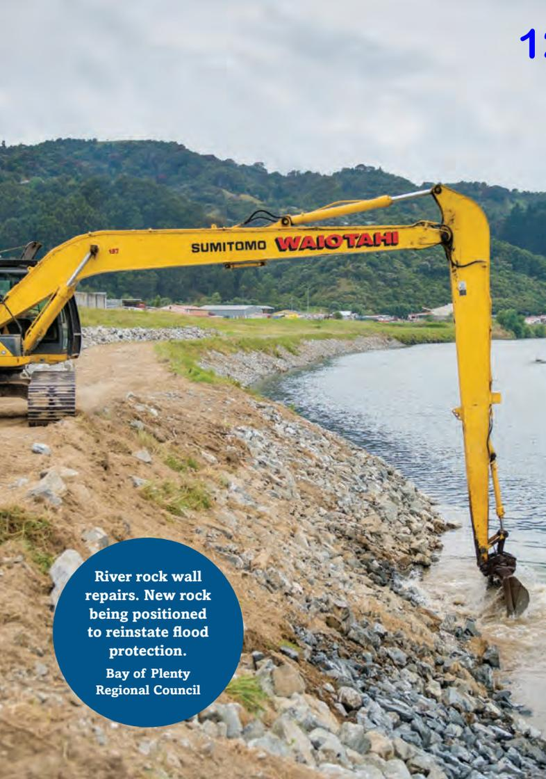
River rock wall repairs. New rock being positioned to reinstate flood protection.
