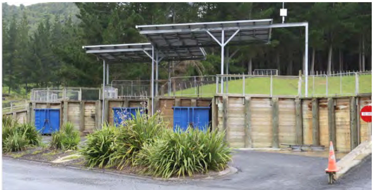
Te Kuiti Transfer Station
