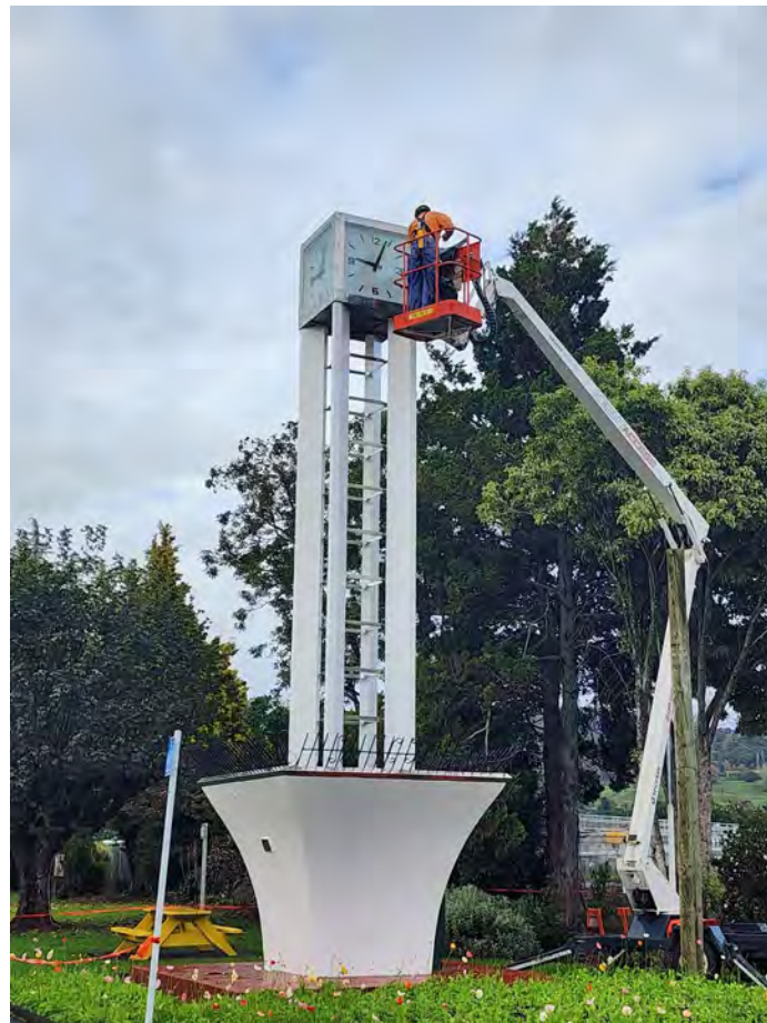
Te Kuiti town clock repair April 2023
