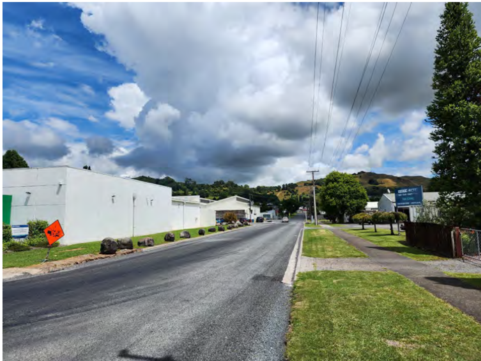
Rehabilitation of Seddon Street, Te Kuiti
