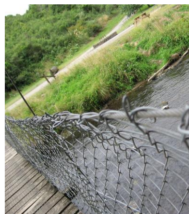
Mangaokewa Reserve Bridge
