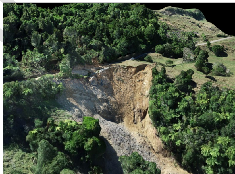
Figure 15: Taumatotara West Road, one of the worst effected roads resulting from Cyclone Dovi (2022)
