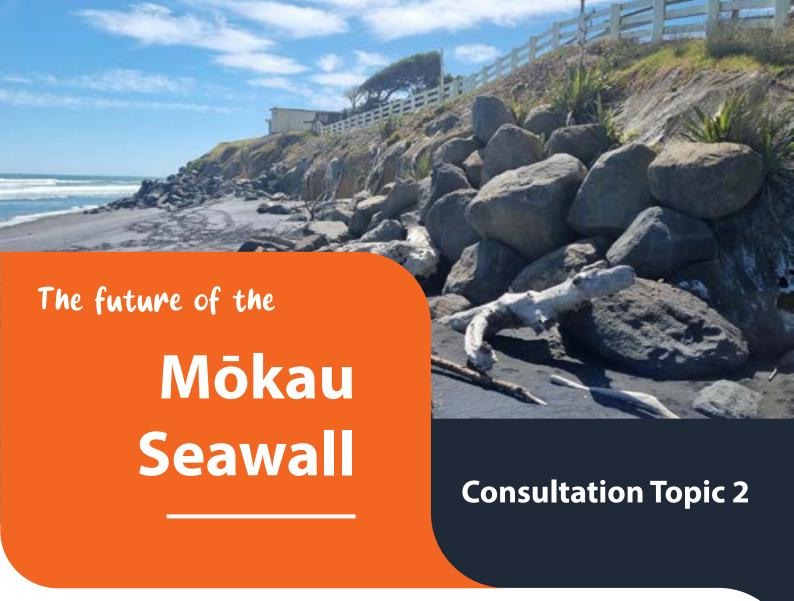
Waitomo District Council built a rock seawall at the end of Point Road, Mōkau in early 2015 to help slow down the erosion of the end of Point Road and retain beach access.
