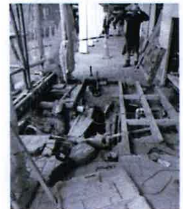
Figure 13 Inner city footpaths in Wellington are narrow and contain more than 100 years' worth of old pipes and cables, making it hard to find a spot for plants.
