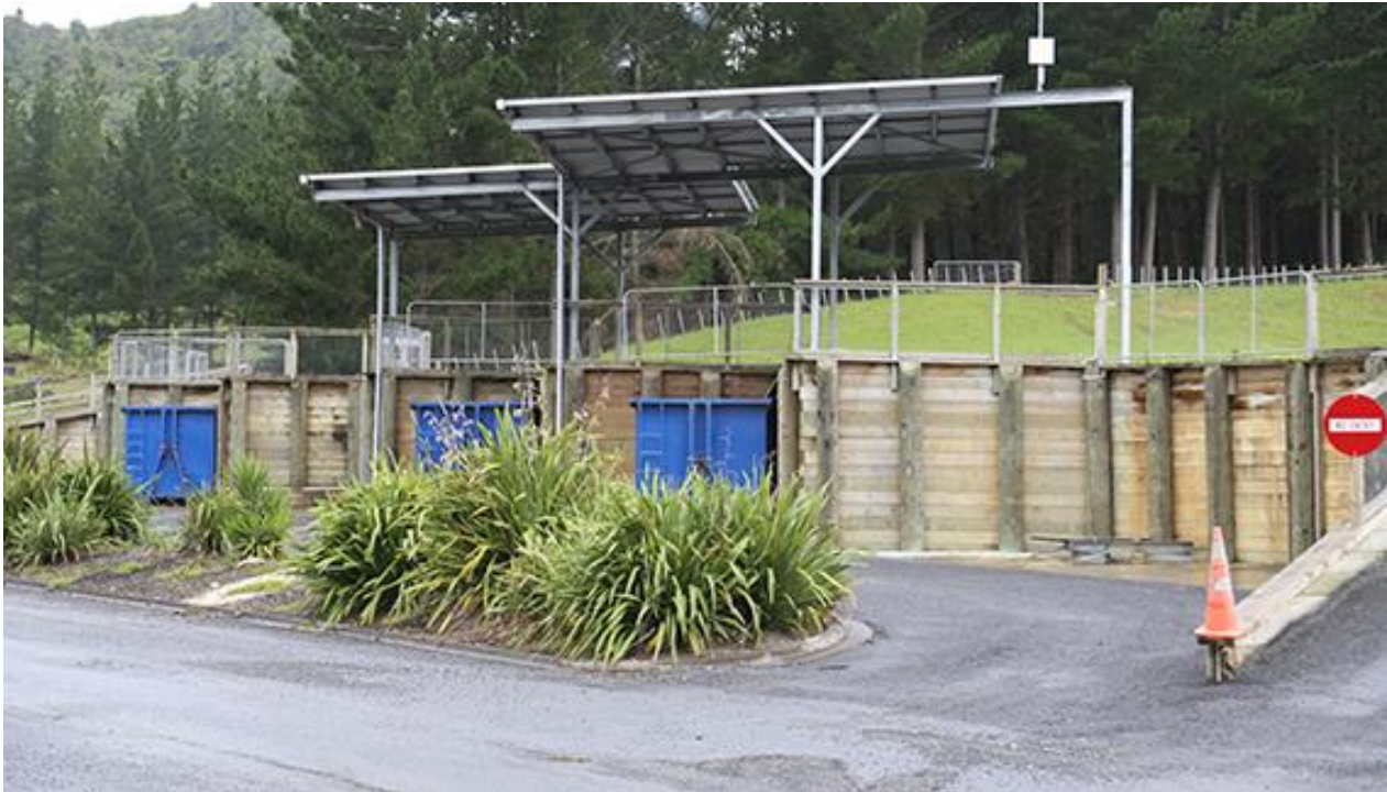
Figure 53 – Transfer station located at Waitomo District Landfill
