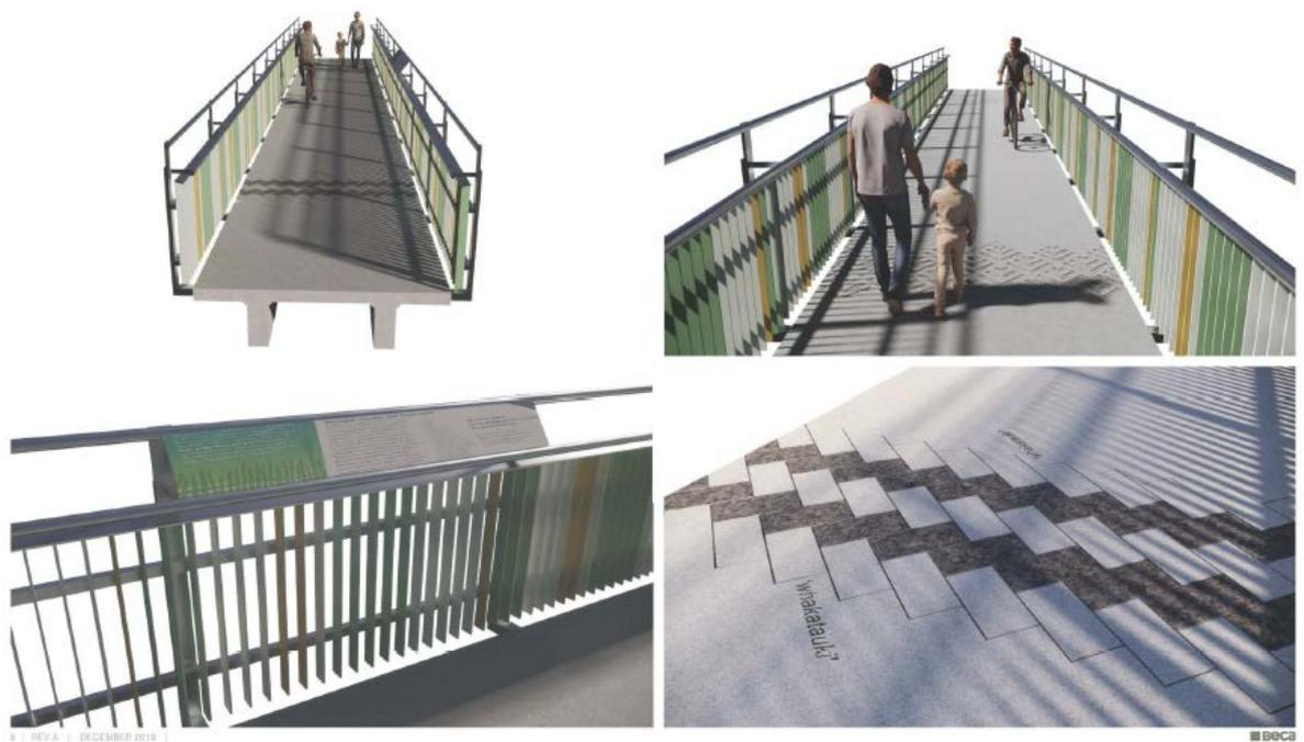
Fig. 11: Architectural elements – Handrails, balustrades, weave patterns and narratives
