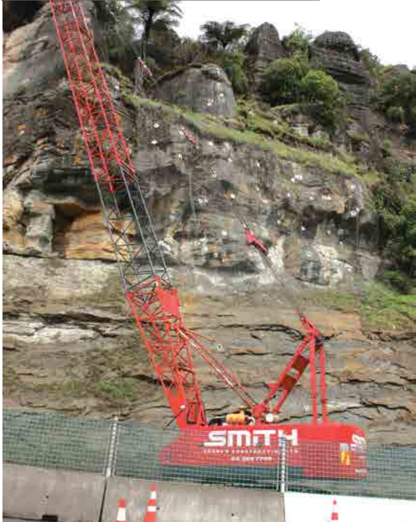
50 DOWN: More than 50 steel rods have been drilled six-metres into the Mangaotaki Bluffs above SH3 as the $2.5 million safety project continues. The stretch of highway has been down to one lane with a temporary barrier to contain rocks following a rock fall in March, killing a Taranaki woman who was a passenger in a vehicle heading north. (Waitomo News, March 28) Another 450 anchors (white spots on the rockface) will be inserted into the rock face just south of Piopio enabling a 1600sq m steel net to prevent further danger to drivers in time for Christmas traffic.
