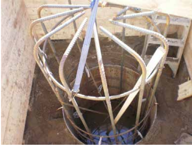
Below – pile foundations designed to soil conditions in this case 20m deep at the Christchurch airport
