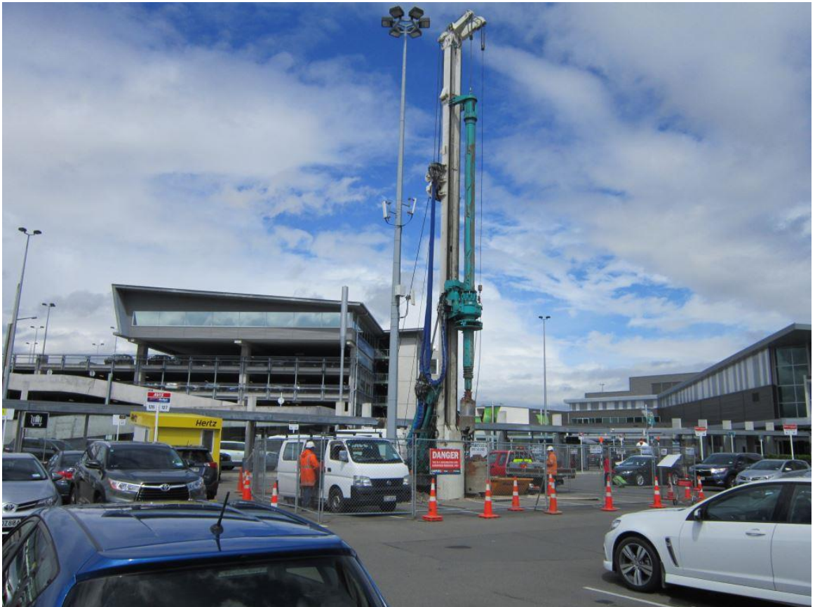
Below – pile foundations designed to soil conditions in this case 20m deep at the Christchurch airport
