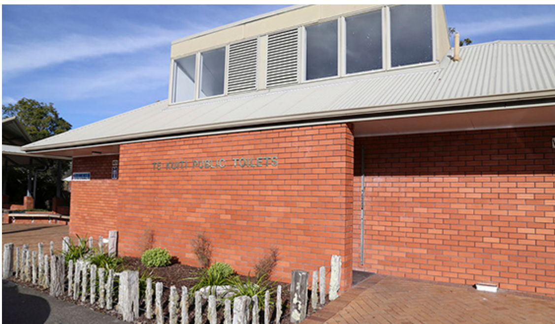
RORA STREET PUBLIC TOILETS
