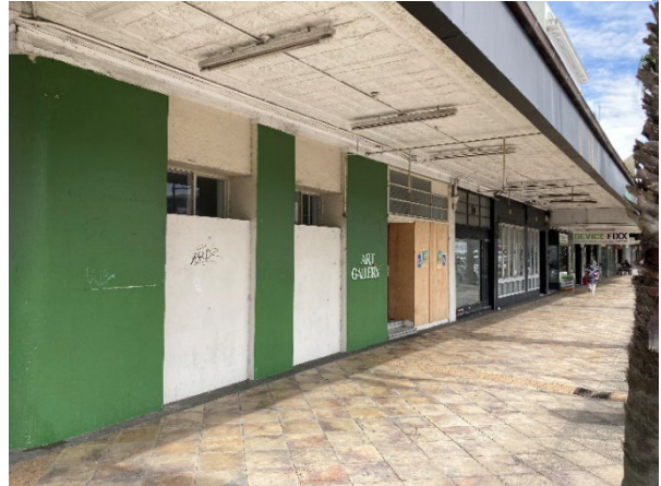
Masonic Hotel frontage. Gladstone Rd
