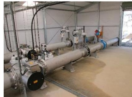
Wastewater Treatment Plant Bulk Lime Silo project has replaced the lime dosing hopper and dosing system, pipework is installed and SCADA integration complete. Dosing will minimise potential health and safety issue.
