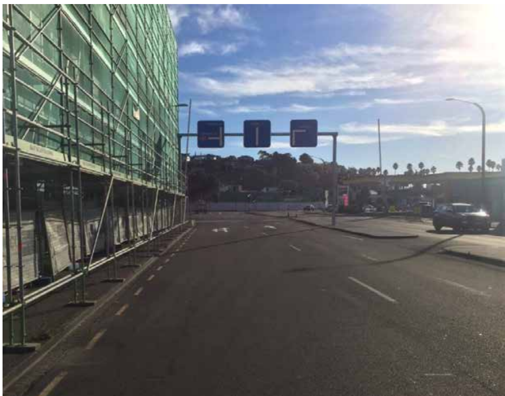
Figure 5 Scaffold obscuring signals for road traffic at a level crossing – view from the road
