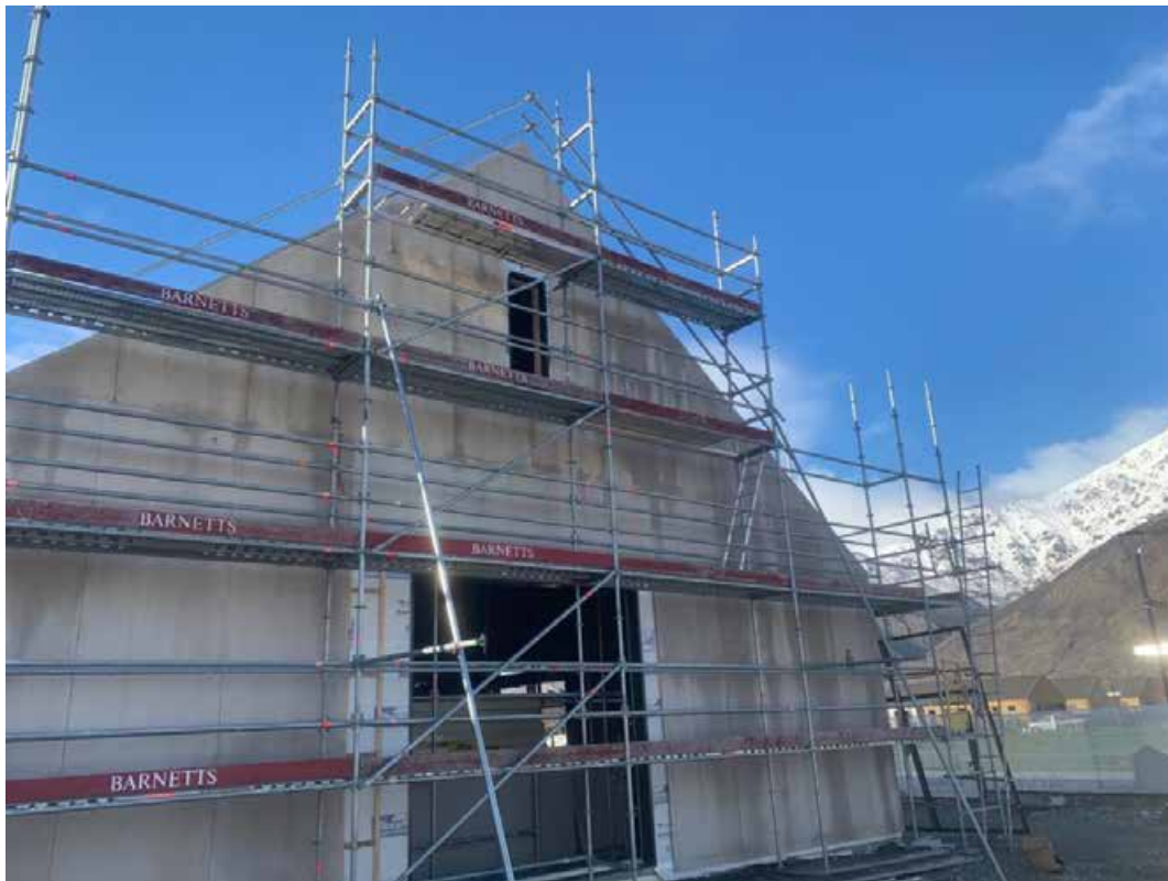
Figure 7 Photograph scaffold with outriggers, credit: Wain Chambers
