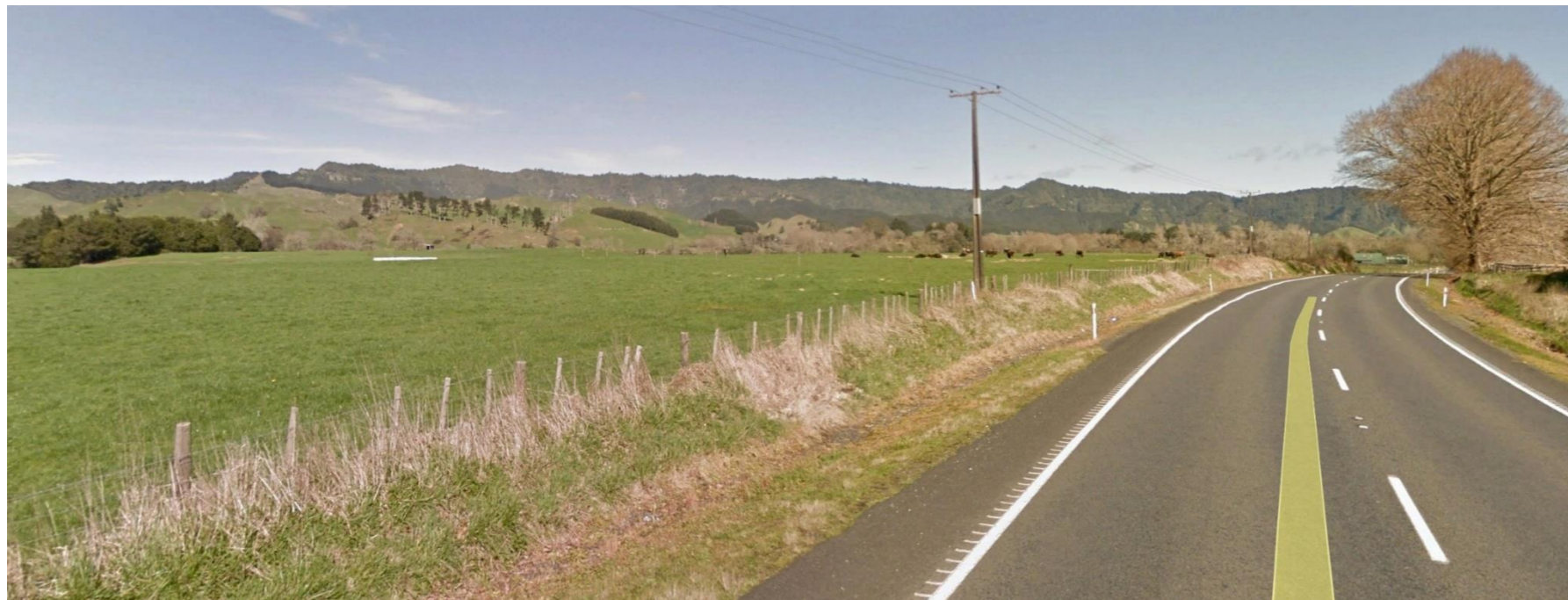
Photograph 111: Typical working rural landscape character straddling SH3 within the unit. LCU 10 Central Rolling Lowlands in midground with LCU 6 Mokau Hills forming backdrop. Source: Google Earth.
