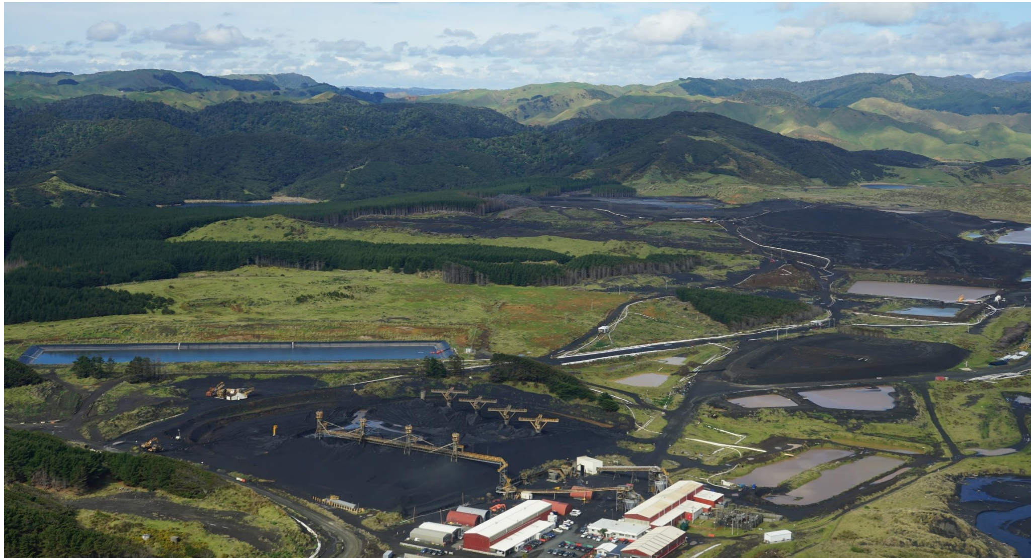
Photograph 48: Coastal hills framing the Dune Lakes with Taharoa Ironsands in the foreground of view.
