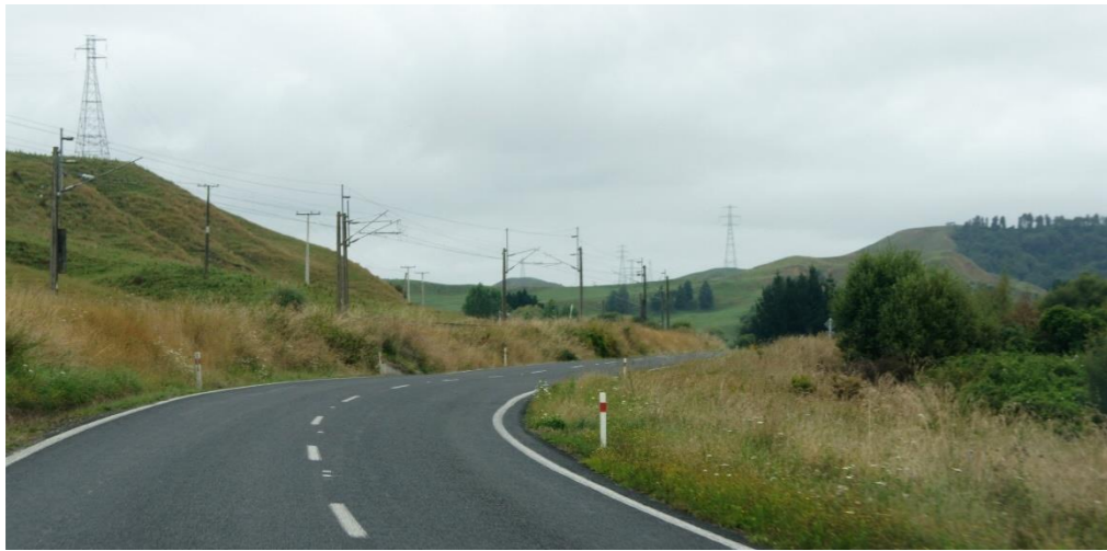
Photograph 121: Transmission line and rail corridor in the unit.
