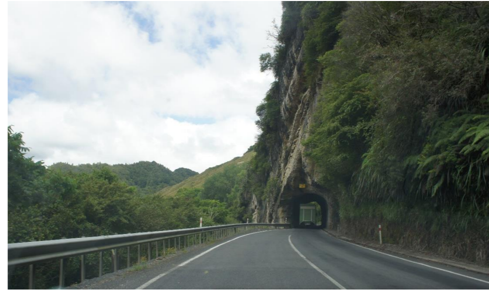
Photograph 83: Awakino Gorge tunnel.
