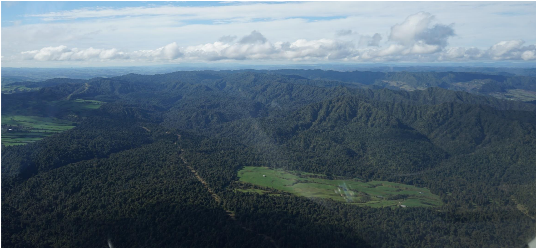
Photograph 75: Typical character of extensive bush clad hill country of LCU 6.
