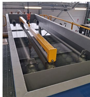
The new membrane unit is lowered into place.
