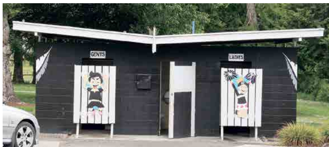
SITTING PRETTY: The brand new public toilets on SH3 in Piopio, which opened last week (above) are designed to cater for large numbers of visitors and replace the old toilets (right) which are being demolished.
