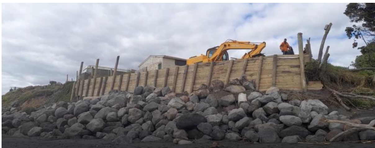
Figure 6 Digger undertaking work to complete retaining wall at end of Council laneway and across northern boundary of burial reserve, Te Naunau, Mokau, October 2022. (Source: M Gibbs collection).
