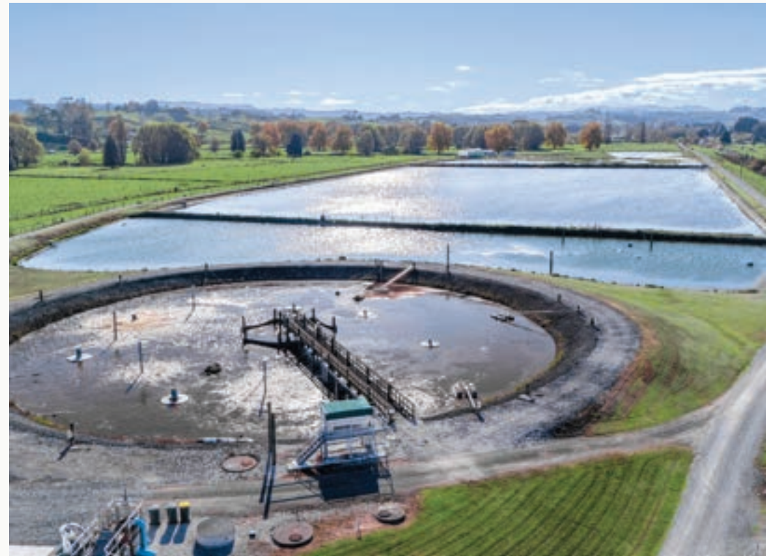
A wastewater treatment plant in Te Kūiti that transferred to Waikato Waters.
