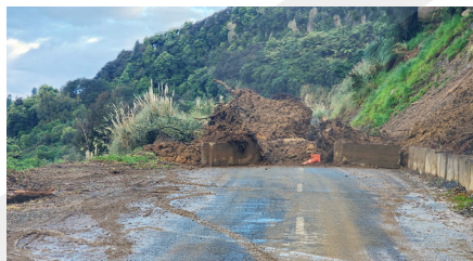
Pukerimu Road slip
