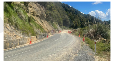
Pukerimu Road cleared
